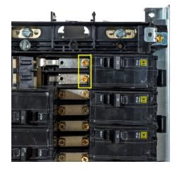
**Step 7** (for QOB Bolt-On Breakers) Using the **#2 square driv**e, tighten down the brass screws to **22 in-lb**.
